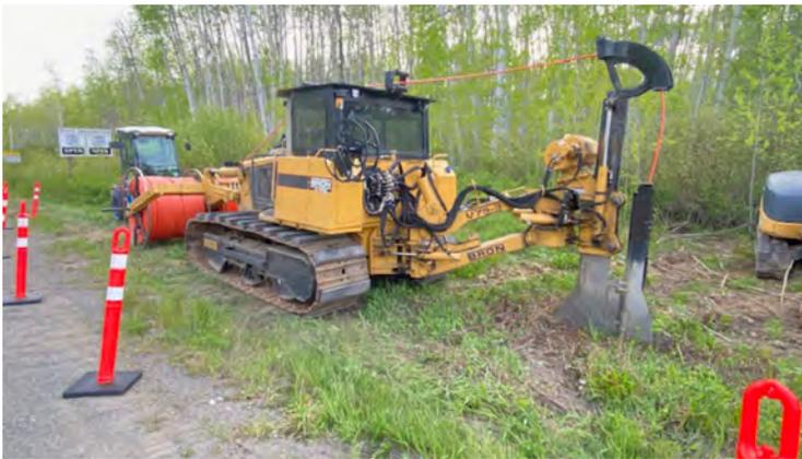
*Above: Installation of 200 kilometres of fibre optic cable to connect Dease Lake and Iskut with highspeed internet construction gets underway north of Kitwanga on Highway 37N on May 31, 2022.*
